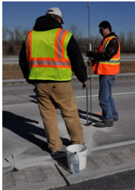
Figure 52. Dynamic cone penetration (DCP) test
