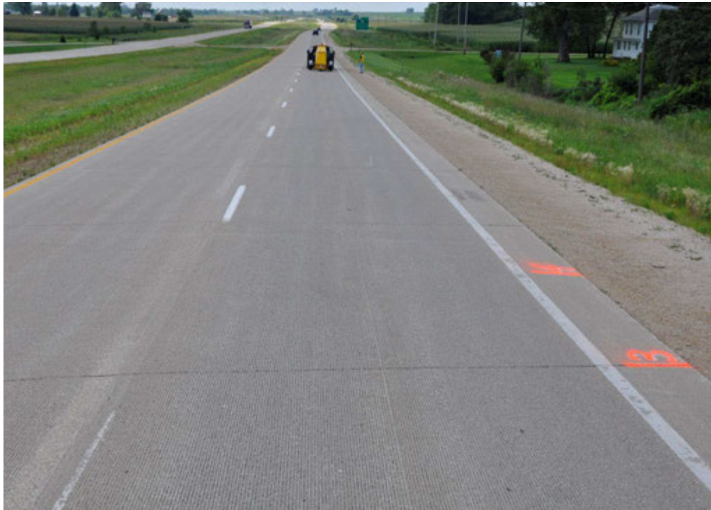
Figure 240. U.S. Highway 218 Plainfield, IA
